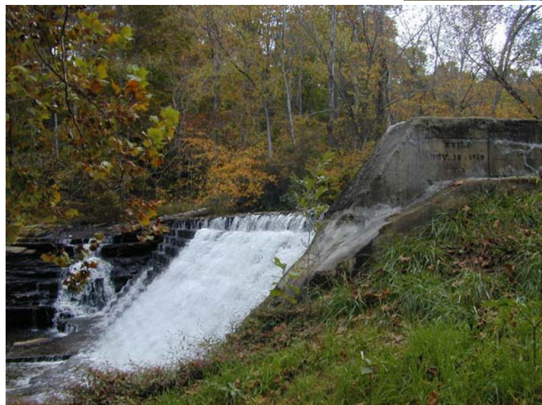
Muddy Creek Mill dam and spillway.
