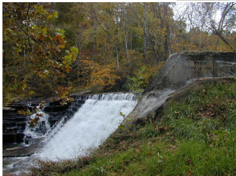
Muddy Creek Mill dam and spillway.
